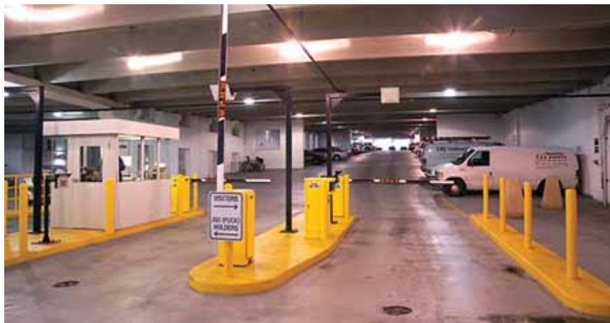
Everything in the lane can be converted to wireless. Many revenue control companies' products can be converted by a system integrator to wireless. Check with your manufacturer to be certain.
